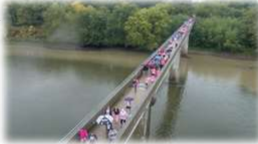
Runners/Walkers crossing Krieg Crossing Bridge
